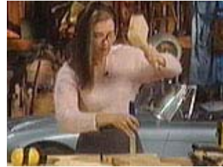
Use a chisel to cut the end of the slot
