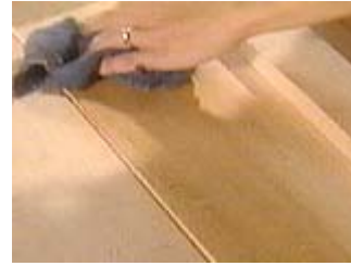
Wipe off excess with a rag
