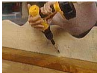
Attach the undercarriage assembly to the finished bench seat
