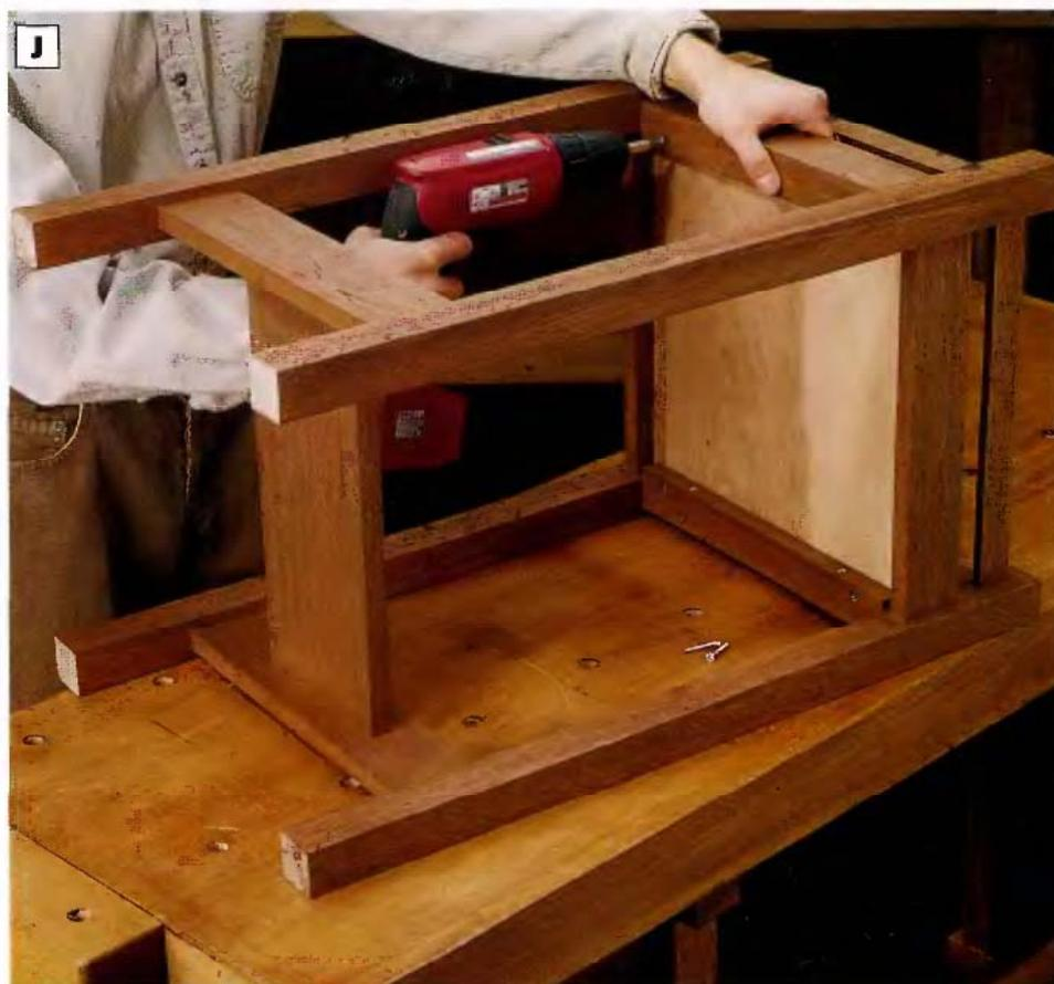
**PHOTO J:** Lay the plant stand on its side and attach the finished tray by driving #6 × 1-in. screws up through the countersunk screw holes in the bottoms of the tray cleats.
