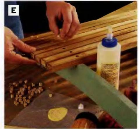
**PHOTO E:** Cover exposed screw heads on the slats and crossbars with oak plugs. Glue and insert the plugs, trim them and sand smooth.
