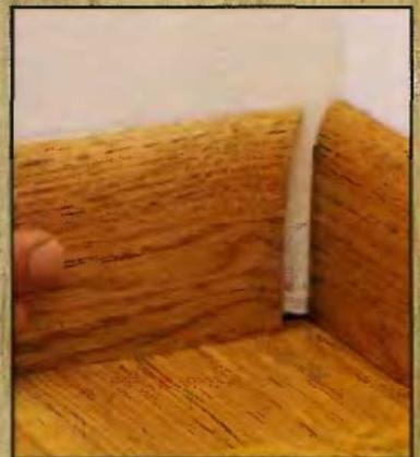
**3** Apply the wood finish to both boards, then slip the beveled board into the corner so it overlaps the end of the square-cut board.
