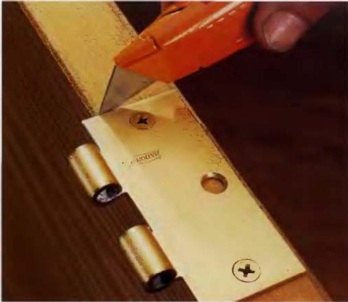
**1** Remove the hinge pin (if its removable) and position the hinge leaf or strike plate on the edge of the door or on the door jamb. Tack it into place with screws, then score an outline around the plate with a utility knife. This prevents the wood from splintering past the ends of the mortise.
