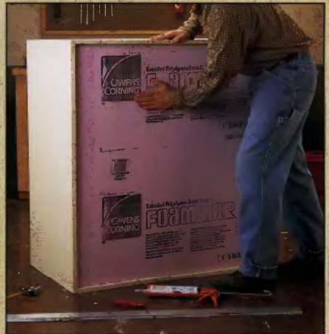
This doghouse project was designed to accept a sheet of 1-in.-thick rigid foam insulation below the bottom panel. Rigid foam is a good choice because it is relatively inexpensive and unaffected by ground moisture. Measure and cut the insulation with a utility knife. Glue it in place with construction adhesive.
