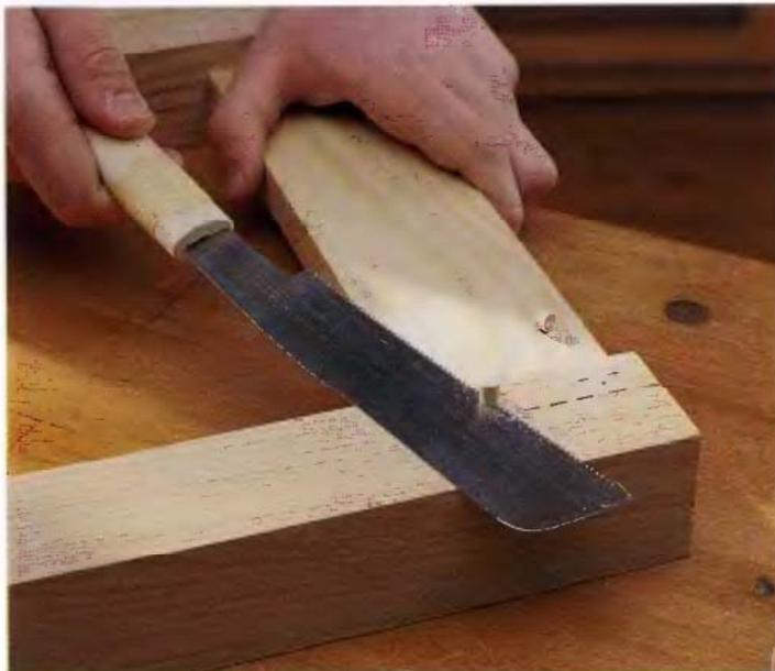
**4** Trim the dowels flush with the leg surface—here we use a flexible, fine-tooth Japanese-style saw. Depending upon the amount of dowel you need to remove, you may be able to smooth the ends flush with a file instead of sawing them off.
