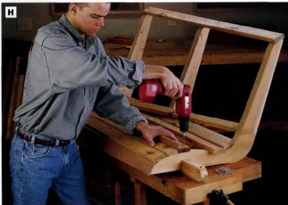
**PHOTO H:** Screw the slats to the back-seat support structures. Butt the first three slats together, then use a ¼-in.-thick spacer between the rest of the slats for consistent gaps. Keep the ends of the slats flush with the sides of the supports.
