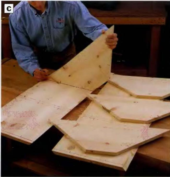
**PHOTO C:** Lay out all the carcass parts and draw alignment marks for biscuit joints. Be sure to keep the orientation of the side panel bevels in mind when you lay out and mark the parts.
