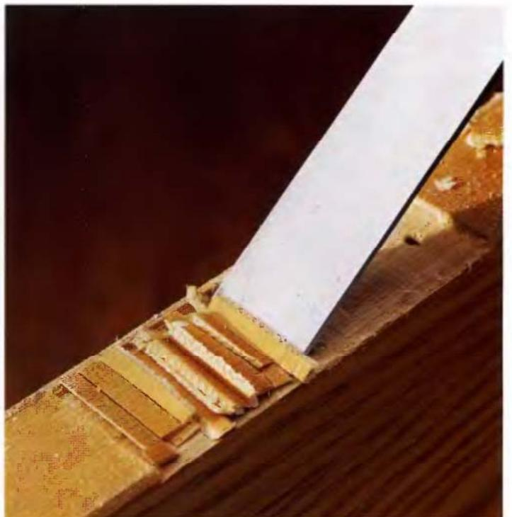
**4** Clean out the waste wood by driving the chisel against the direction of the relief cuts. To avoid digging in too deep, try to keep the beveled edge of the tip flat in the mortise. Scrape the bottom of the mortise smooth. If you need to deepen the mortise, repeat the procedure—don't simply try to make deeper scraping cuts.
