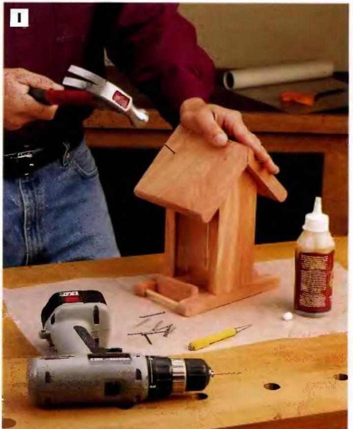
**PHOTO I:** Attach one half of the roof to the body of the bird feeder with polyurethane glue and galvanized 4d nails. The other roof section hinges open to allow easy access for filling and cleaning the feeder.
